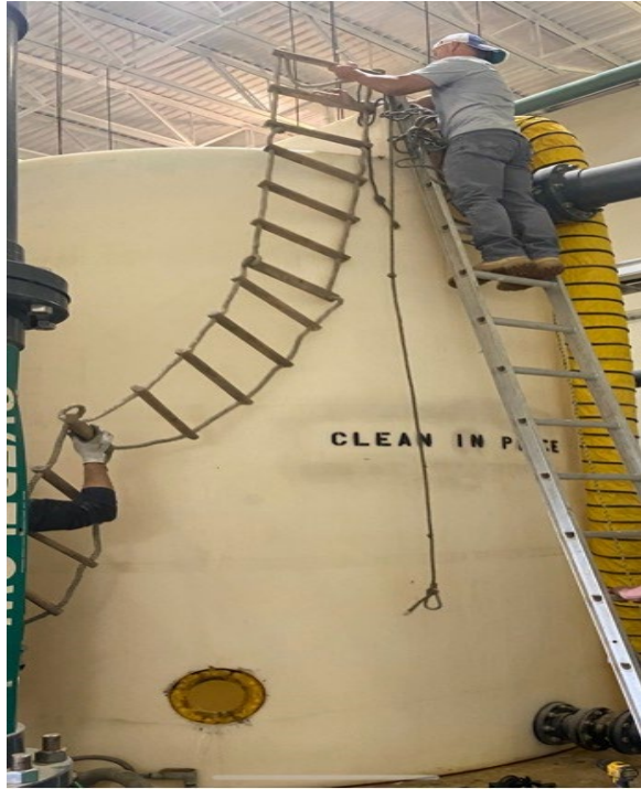
*Pictured above left, Plastek Werks prepares for welding CIP tank.
