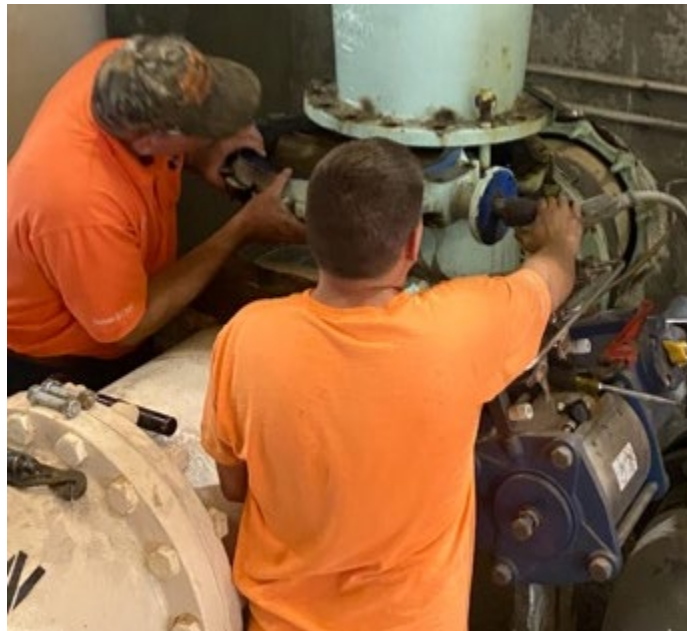
*Pictured above, CC&A installs new 16” fill valve on train 1.
